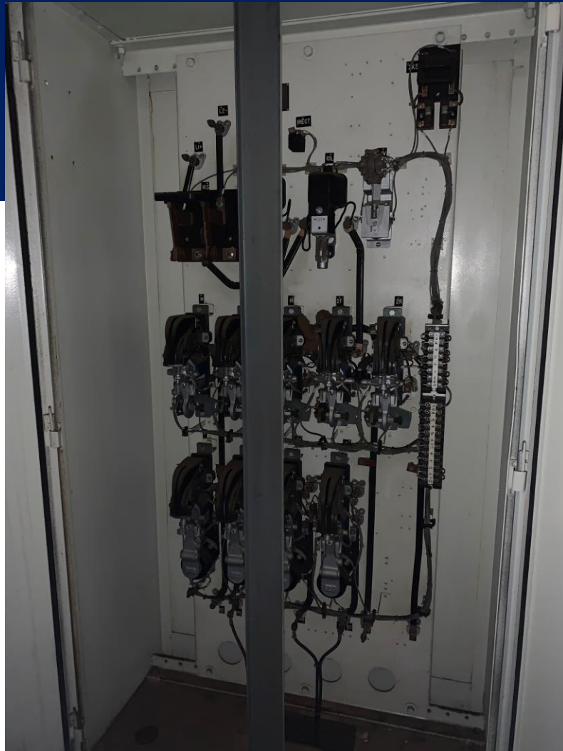
(2) Nema Size 3, 10 HP, 230 Volt DC, Cutler Hammer Trolley Control Panel, Front Wired, 5-Speed, 900 Series Contactors, mounted in Enclosure, complete with resistors mounted in fabricated steel racks
